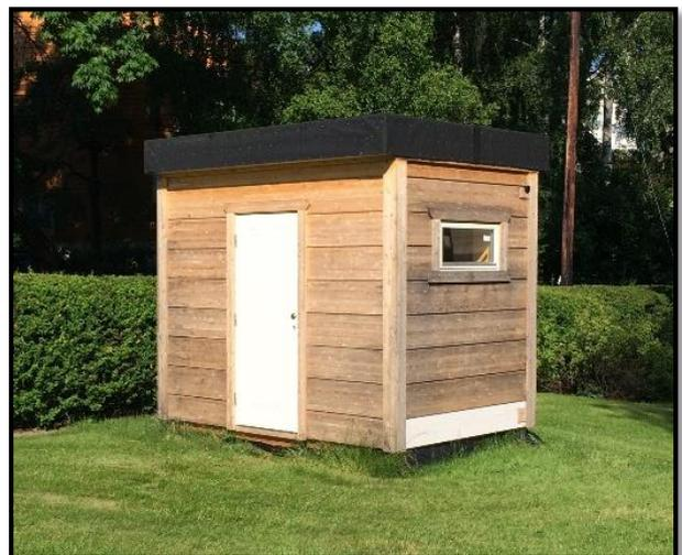
**Figure 1:** Exterior view of the testhouse built of the wood-based insulating sandwich panel
